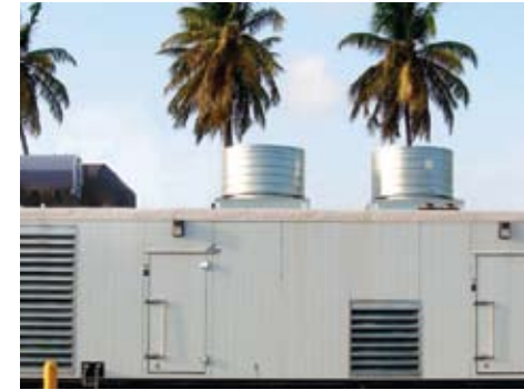
Enclosed gen set providing back-up power for a resort on the Caribbean Island of St. Kitts
